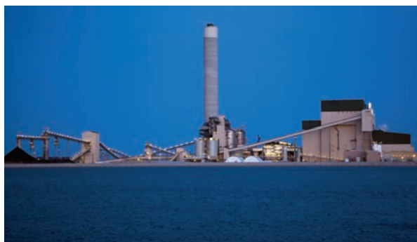
The first unit of the Prairie State Generating Company began commercial operation in June 2012.
